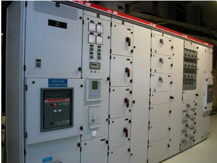
*The short circuit currents are lower with 690 V voltage. This affects the construction of the switchgear, which is smaller today than before, and facility space can be used for other purposes.*
