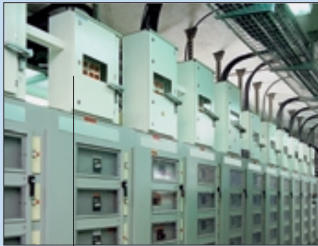
Safety breaking enclosures placed for each incomer: additional safety for maintenance operations on the distribution pillar.
